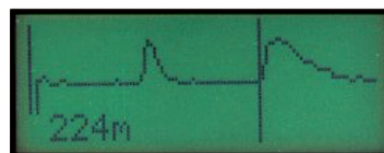
Graphical display of cable faults with digital indication of distance
